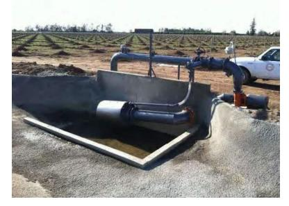
Figure 3. Alternative turnout structure to allow direct pumping from district canal to supply an onfarm pressurized irrigation system. During and following construction.
