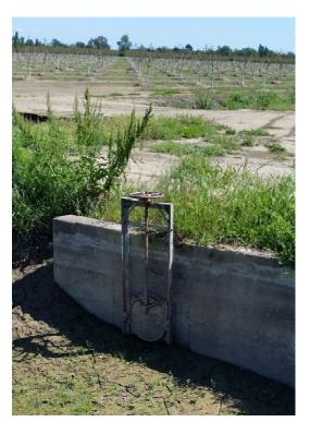
Figure 6-4 Canal Turnout Gate without Trash Rack or Screen
